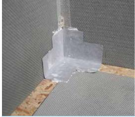
Use 'Marmox Acrylic Sealant' to fix 'Marmox Waterproof Corners' into position. Make sure to push fully into the corners.
