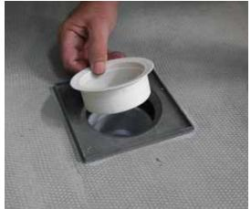
Place the plastic ring through the hole and into the drain.
