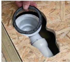
**8** Cut out the key hole shape drawn and place in drain. Connect with pipework using a solvent weld. Then place the rubber ring onto the top of the drain.
