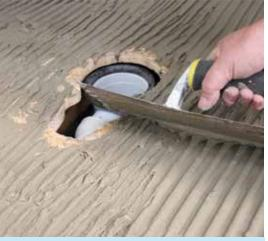
Using a full bed of flexible cement based tile adhesive, fix the Showerlay to the floor. Continue checking it is level in all directions.
