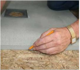
**2** Be aware of where the floor joists are and position the Showerlay with the hole inbetween them. Then draw around the edges of the wooden floor using a pencil.
