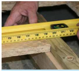
4 Lower supporting shelves between the joists (minimum of 18mm). Make sure that the support is flush with the joists and fully supporting. Be aware of floor level.
