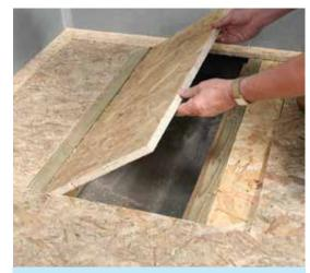
**5** Place the support into position and check again that the floor is level in all directions.
