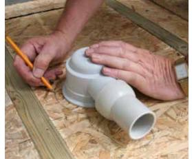
7 Sit the drain upside down over the pencil mark. Now draw a further pencil mark around the Dallmer drain (plus 10mm). Allow room for the drains knuckle.
