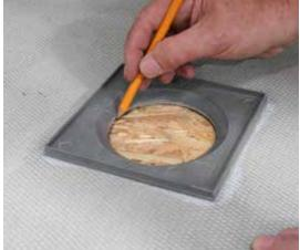
**6** Lay the Showerlay down onto the supporting shelves and mark out the hole position with a pencil.
