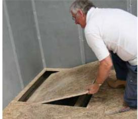
**3** Cut out the floor the section using an electric Jigsaw.
