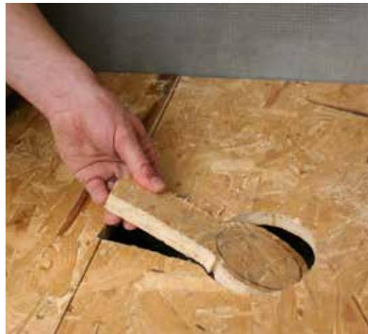
**3** Cut out a hole big enough to fit the Dallmer drain. This should be slightly larger than the mark made on the floor and should allow room for the Dallmer drains knuckle.
