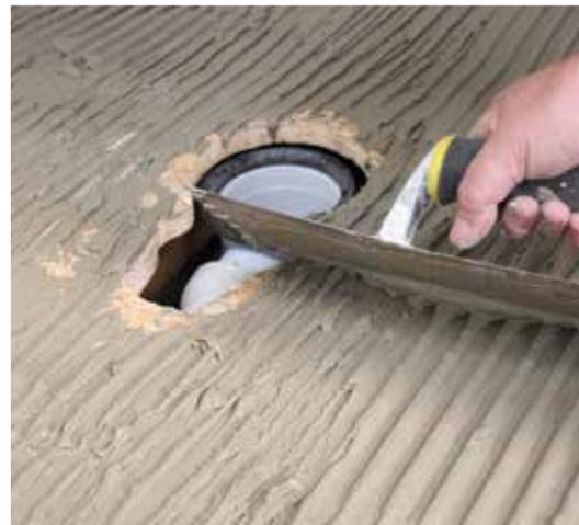
**7** Using a full bed of flexible cement based tile adhesive, fix the Showerlay to the floor. Continue checking it is level in all directions.
