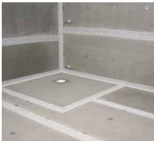
**15** Tape around the main wet areas with Marmox Self Adhesive Waterproof Tape. Now tiling can begin directly onto the Marmox.
