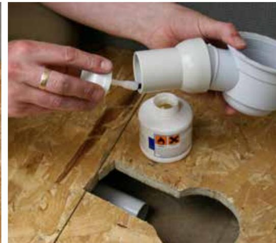
**4** Position the pipework. Make sure the Dallmer drain lines up correctly and then connect the pipework to the Dallmer drain using a solvent weld.
