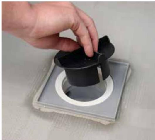
**10** Using the tool provided, screw the plastic ring as tight as possible.
