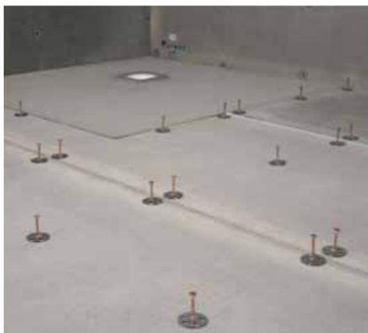
**14** Using 20mm Marmox boards, cover the rest of the floor. Fix down using a good quality cement based tile adhesive or screws and washers at every 30cm.
