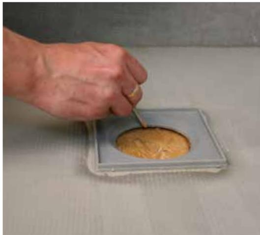
**2** Mark out the drain position on the floor.
