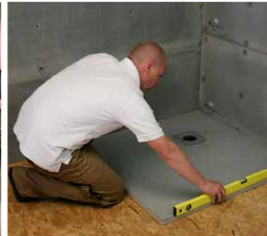
**8** Push the Showerlay down firmly to the floor and then check again to make sure all is level and there is no movement at all.
