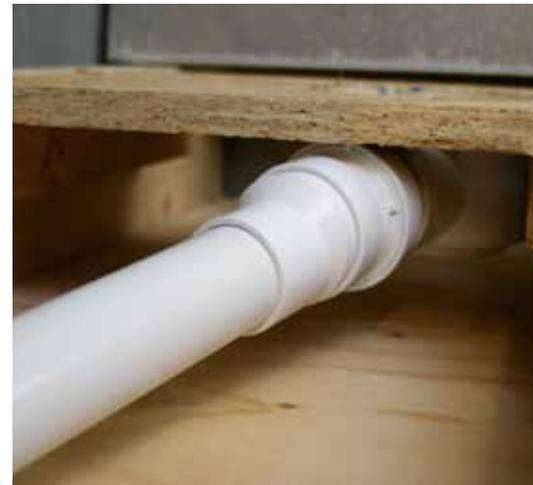
**8** Fix to the main drain pipe (BS 40mm) and make sure the drain pipe slopes away from the drain to allow proper drainage.
