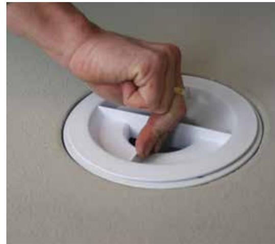
**12** Screw the drain collar through the Showerstone drain hole into the gully. Use the circular plastic key supplied to tighten it as much as is possible.
