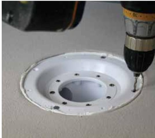
**13** Drill through the plastic collar and metal plate, into the support shelf (3mm metal drill). Use a 20mm screw. Repeat this for the other 3 indents in the plastic collar.
