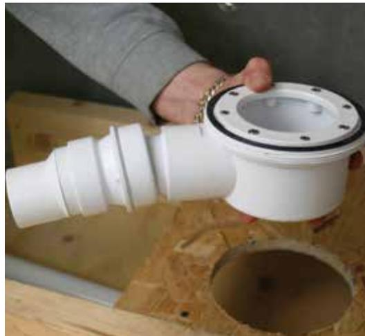
**7** Fix the drain pipes together (see the McAlpine drain instructions for full details).
