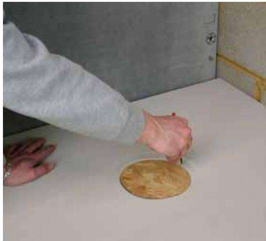
**5** Mark out the drain area on the support shelf by penciling around the edge of the hole and then cut out a hole in the shelf.
