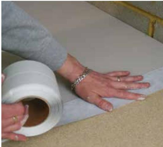
**14** Use Marmox Multibond and, if tiling Marmox Waterproof tape, around all the edges and up the corner of the wall.
