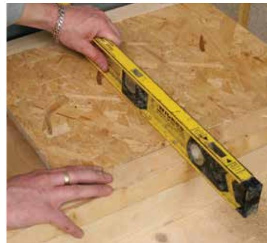
**4** Make sure support is flush with the floor joists and that all floor joists are level. Maximum joist span is 450mm.
