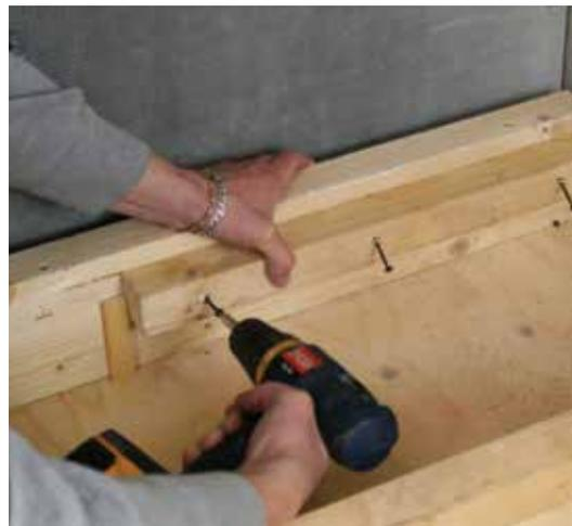
**3** Use part of the removed floor-boards, or 18mm timber, to create a shelf, between the two joists under where Showerstone's metal plate and drain will sit.
