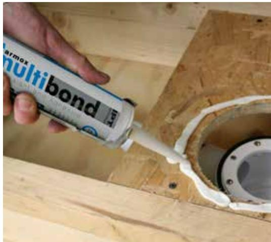
**9** Use Marmox Multibond on the support shelf and a generous amount along the floor joists.
