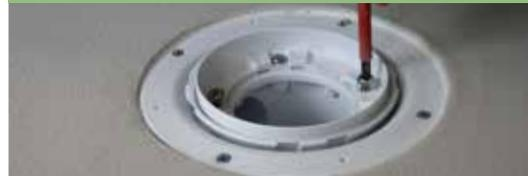
**15** Screw in the drain ring (and optional extension) and place the hair trap inside.
