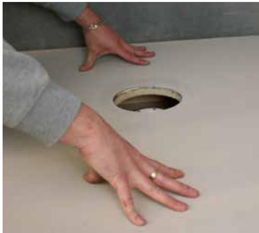
**10** Position the Showerstone into place and press down firmly. Using a masonry drill and 40mm screws, fix the perimeter to the joists at every 300-400mm.
