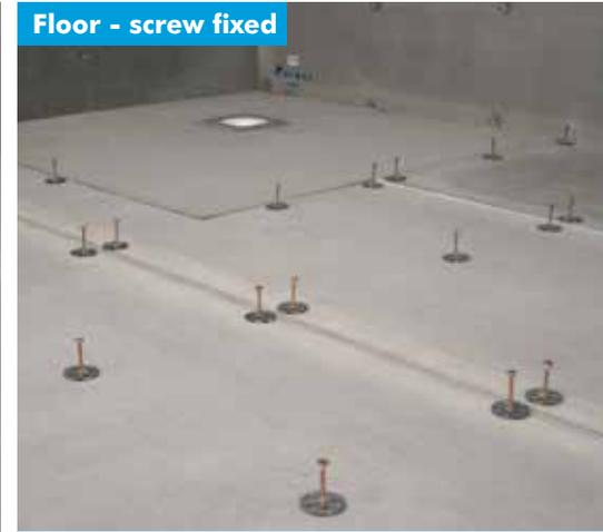
**1** For screw fixing use a screw and Marmox washer at every 300mm.
