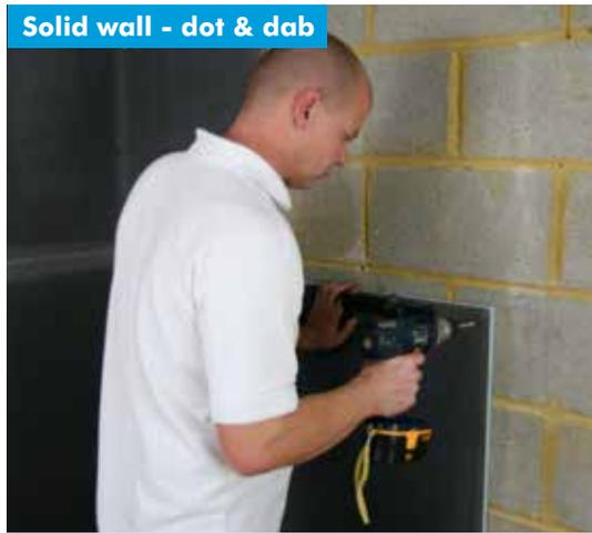
**1** Create 5 fixing holes through the Marmox Multiboard. Minimum board thickness 12.5mm.
