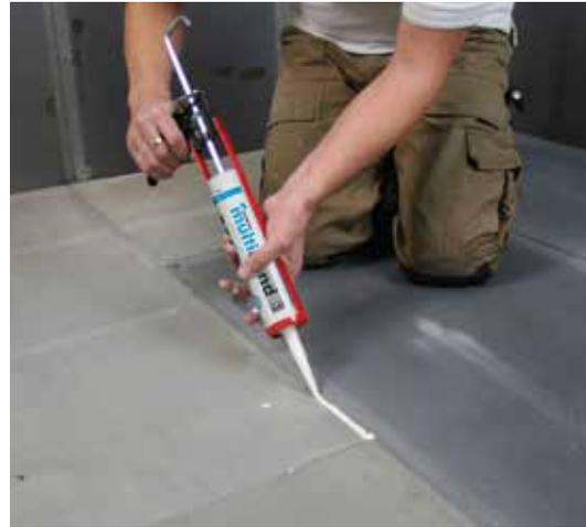
**3** You can use Marmox Multibond for further waterproofing or in really wet areas use Marmox Self Adhesive Waterproof Tape.
