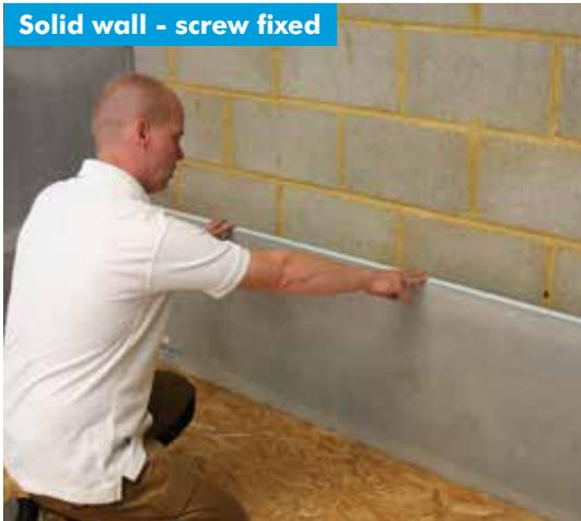
**1** Measure Marmox Multiboards and cut to size. Very easy to cut with a knife or saw.
