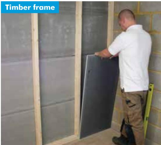
**1** For a stud wall build with 600mm centres, use 20mm Marmox Multiboard or thicker. 10 and 12.5mm thick boards require studs at 300mm centres. All board edges should be supported.
