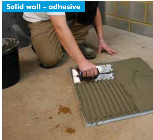
**1** Use a 6/8mm trowel to comb adhesive over the whole surface of the Marmox Multiboard. For uneven walls increase to a 20mm trowel.
