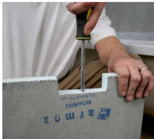
**7** Drive a screwdriver into the panel in the centre of the cut out section to allow the bolt to sit inside the foam.
