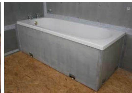
**16** You can waterproof where the bath panels meet the wall with 'Marmox Acrylic Sealant' if desired. Also 'Marmox Self Adhesive Waterproof Tape' can be used to make all edges fully waterproof.
