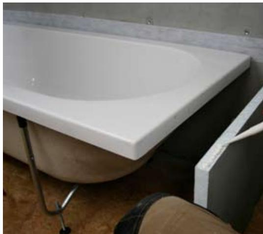
**9** Apply Marmox Acrylic Sealant all the way along the top of the end panel.
