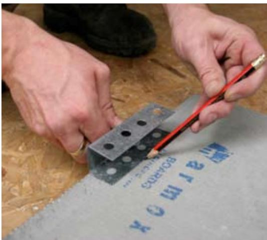
**5** Hold the feet against the bottom of the end panel and mark around it. This should be roughly 100mm in from each end. 2 feet per panel
