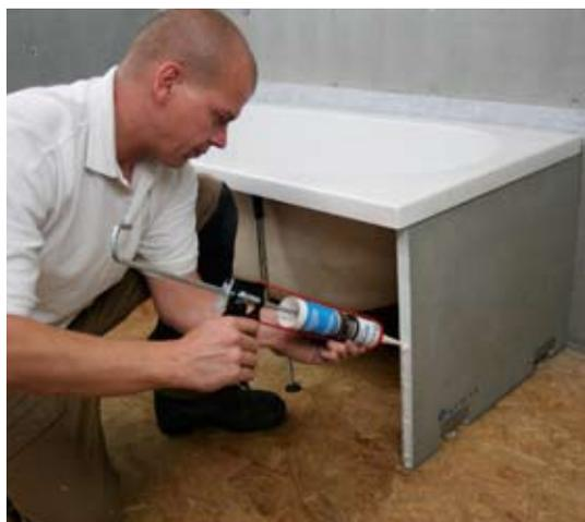
**13** Prepare the side panel in the same way by cutting it to size and adding the feet. Then run a bead of Marmox Acrylic sealant up the side of the end panel.
