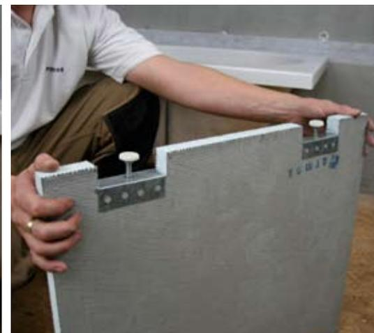
**8** Push fit the feet into position and screw the feet down until they are flush with the edge of the board.
