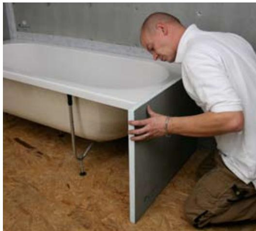
**3** Measure and mark the smallest panel against the end of the bath. Be sure to leave a 30mm gap on the outer edge for the side panel to sit in front of.
