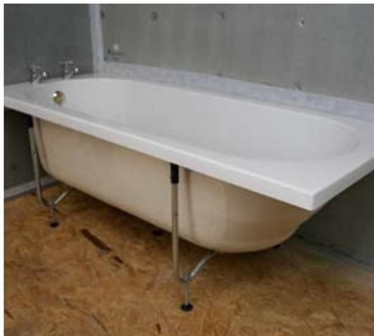
**2** Position the bath and make sure you have enough room to allow a 30mm panel to fit under both sides. Move legs over if necessary.
