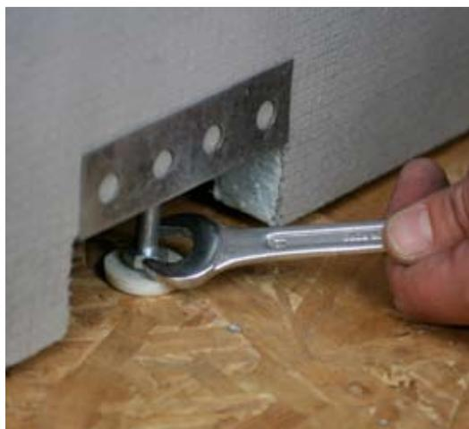
**15** Adjust the feet as is necessary using a 13mm spanner.
