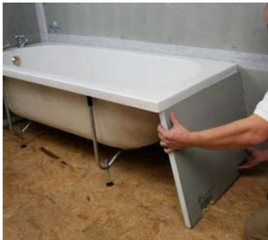
**10** Wedge the end panel under and up into the bottom of the bath.
