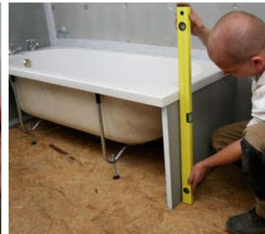
**12** Make sure panel is level and check the 30mm gap allows for the side panel to overlap on the corner.
