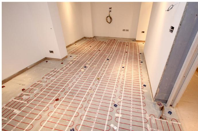
Employing the Marmox Multiboards in two different sizes helped speed the work, while ensuring accuracy, together with long term performance. In total Marmox supplied some 1000 square metres of Multiboard in the 2500 x 600 (Longboard) and 1250 x 600 (Standard board) options; at 12.5 and 6mm thickness respectively.
