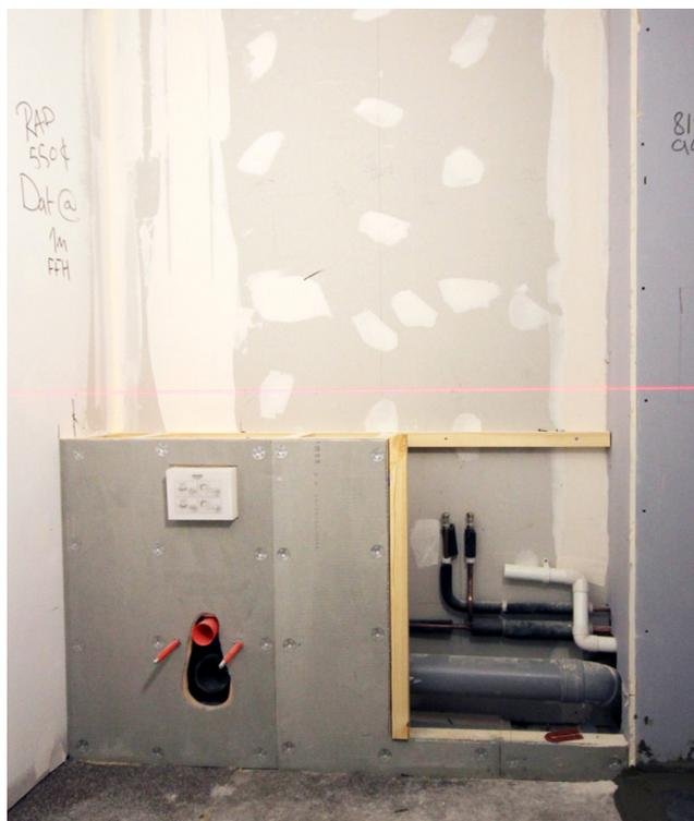
Marmox Multiboards are manufactured from extruded polystyrene or XPS and offer a range of positive physical characteristics in addition to being fully waterproof. They are both light to handle and easy to cut, while still being able to sustain substantial loadings if required. They further offer good thermal insulation performance, helping to cut condensation risk.
