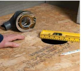
2 Draw a larger circle around the hole with a diameter of between 130mm to 150mm and cut this out using a saw.
