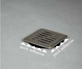
1 Check that the height of grate in the silver frame will be level with the tiles when fixed with adhesive. To secure and stabilise the drain frame, pack some tile adhesive underneath.
