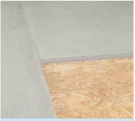
**8** If using a 20mm thick Showerlay, the rest of the floor can be raised to this height with Multiboard 20mm.
